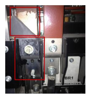
In the example shown to the left, the left bus bar insulation is damaged and the terminal connection pads are discolored.
